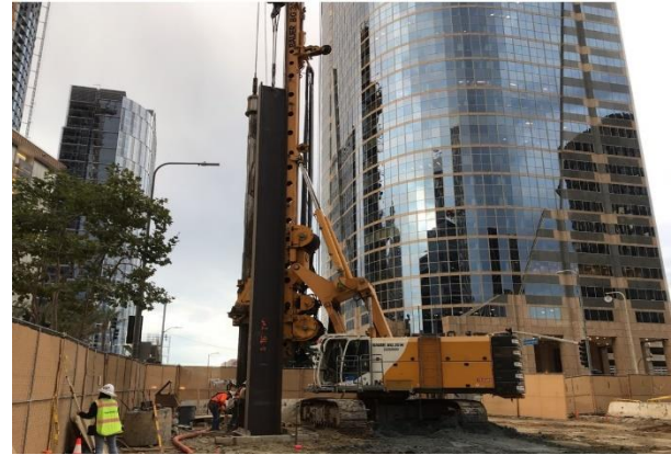
Pile Installation in Century City
