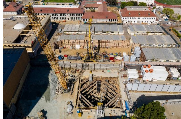
Tunnel Access Shaft in Century City
