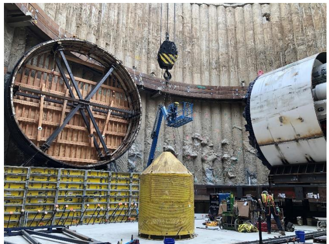
Headwall at Base of Excavated Tail Track Exit Shaft
