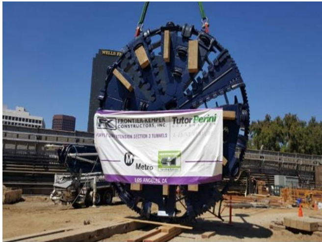
Lowering of Cutterhead in the Tail Track Exit Shaft
