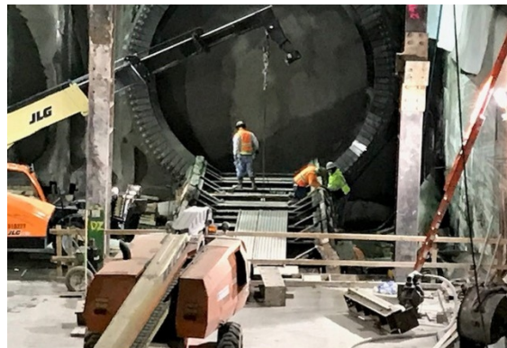
TBM Cradle Assembly at Wilshire/La Cienega Station
