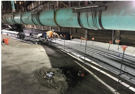
Conduit Installation on Wilshire/La Brea Station Roof
