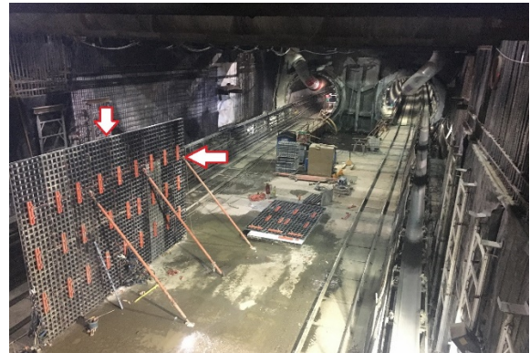
Interior Wall Form Installation at Wilshire/Fairfax Station
