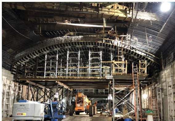
View of Arched Roof at Wilshire/La Cienega Station
