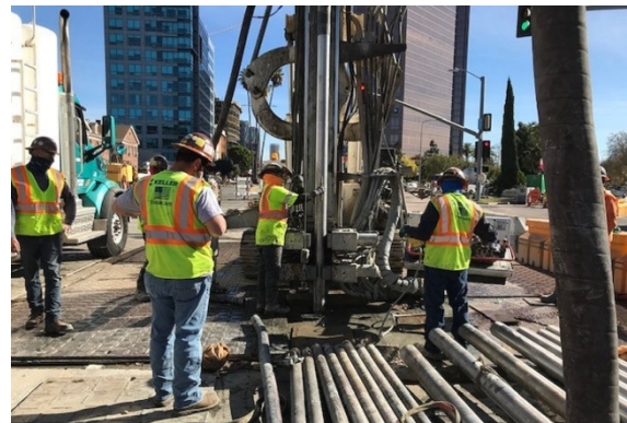
Reach 3 Anomaly Work at Wilshire/San Vicente
