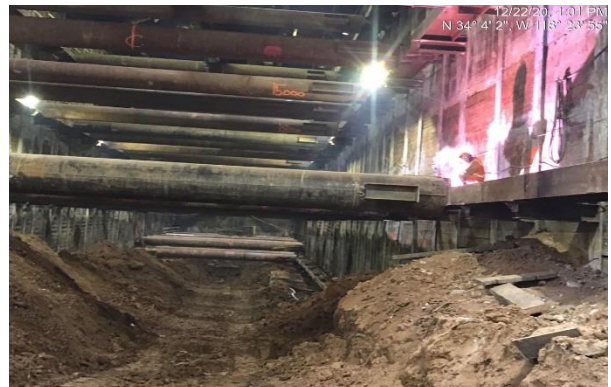
Excavation Activities Wilshire/Rodeo Station
