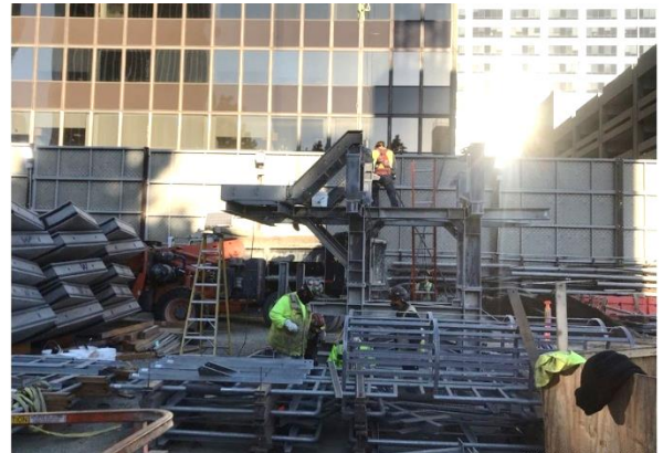
Preparation for Tunneling Transition to Tunnel Access Shaft
