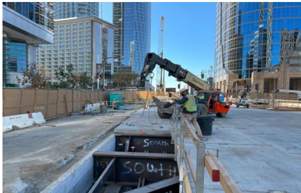
Decking Installation West of the TBM Launch Box
