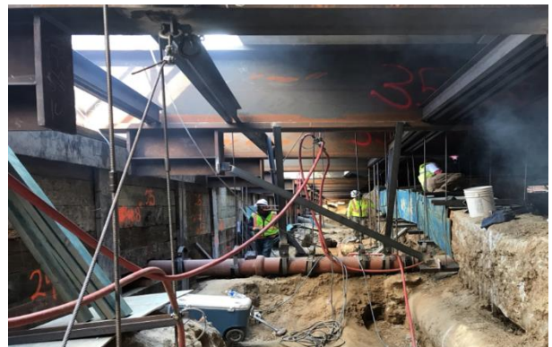
Utility Hanging West of the TBM Launch Box
