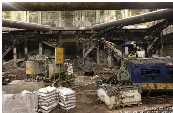
Canopy Pipe Drilling Wilshire/Rodeo Station
