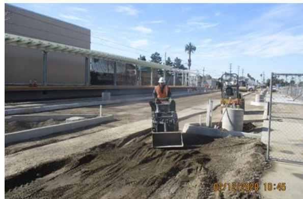
Fine grade for asphalt at Fairview Heights Station parking lot
