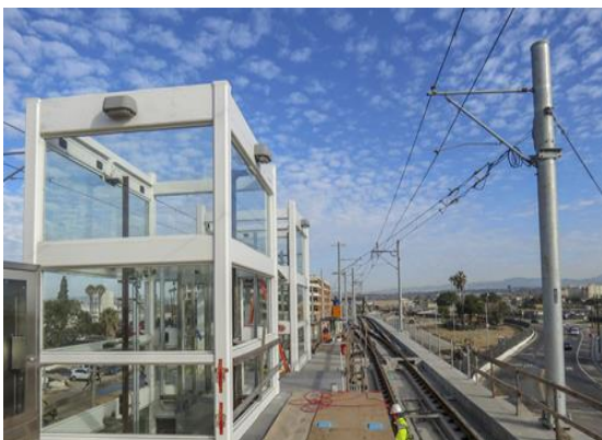
Aviation/Century Station elevator progress
