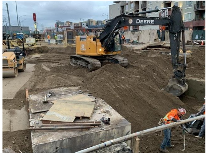
Street restoration at 1st/Alameda
