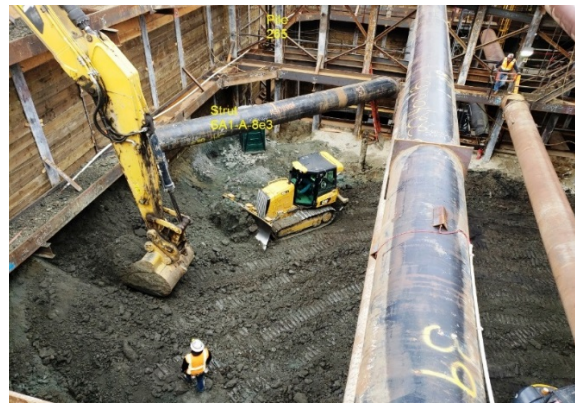
Entrance Appendage Excavation at Wilshire/Fairfax Station
