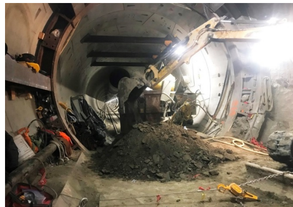
Reach 1 Cross Passage #12 Excavation
