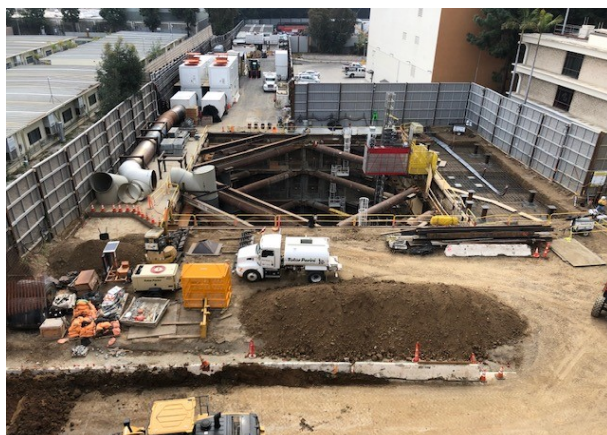
Access Shaft in Century City
