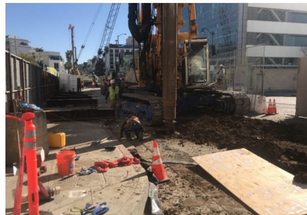
Wilshire/Rodeo Station Pile Installation on Wilshire Boulevard
