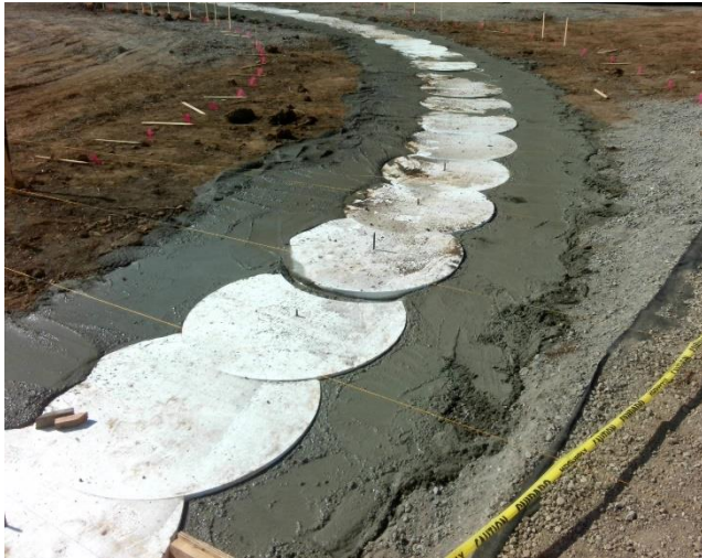
First 100 Feet of Guidewall at Western VA Staging Area
