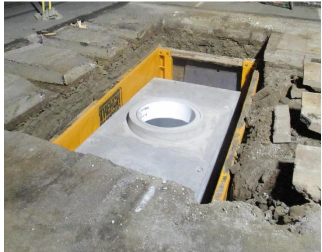
MH 800 on Wilshire Blvd. East of Federal
