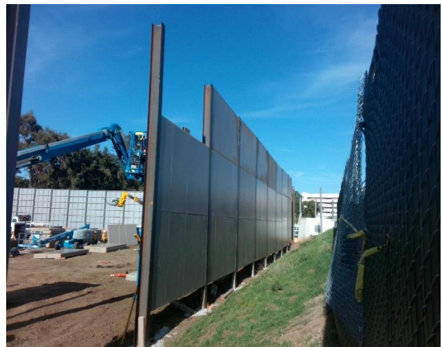
Soundwall Installation at VA Site
