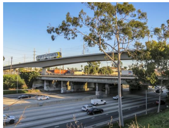
Vehicle testing on new bridge over I-405
