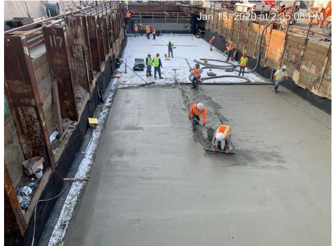
Protection slab placement at 1st St Leg
