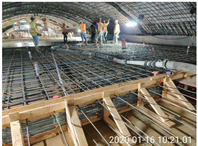
Concrete placement at SEM Cavern plenum
