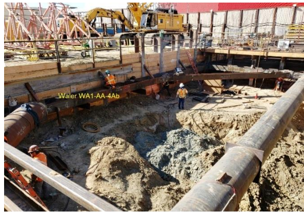
Entrance Appendage Excavation at Wilshire/Fairfax Station
