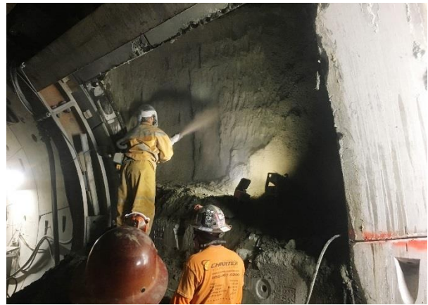
Reach 1 Cross Passage #11 Excavation
