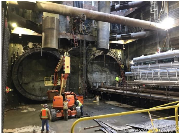
Tunnel Eyes and Gantry at the Launch Box in Century City
