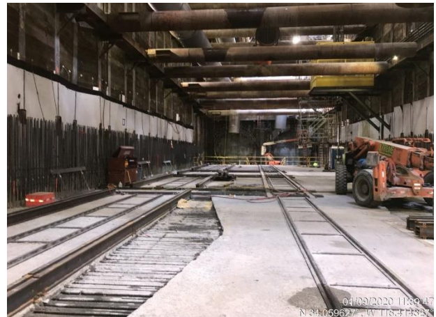
TBM Launch Box in Century City
