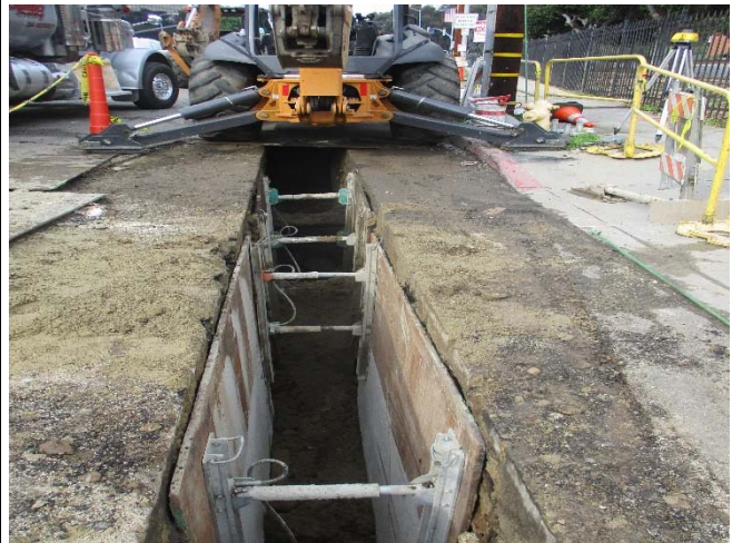
Continued Excavation for SCE Ductbank
