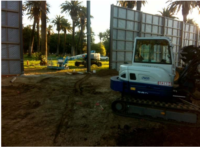
Soundwall Installation at the VA Site
