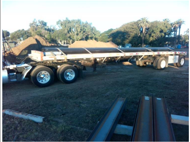
Storm Drain Pipe Delivery
