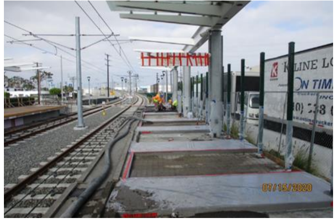
Hindry Station – Placing concrete for topping slab for southbound platform.
