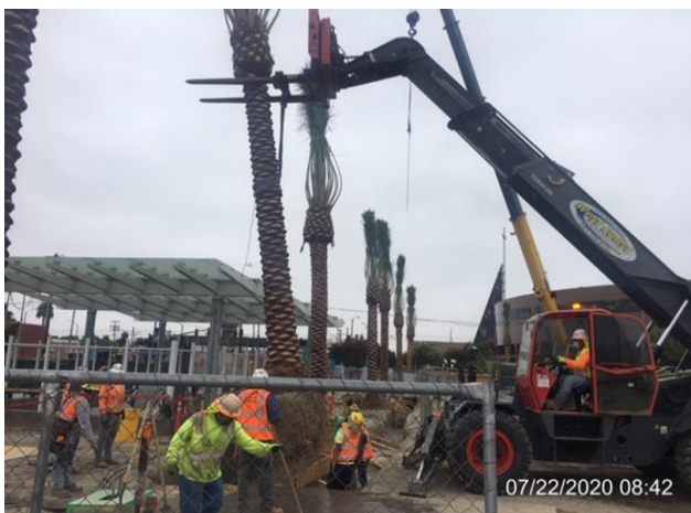
EXPO Station– Continue palm tree installation throughout plaza level
