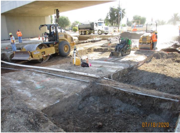
111 th Street – Base placement and compaction.
