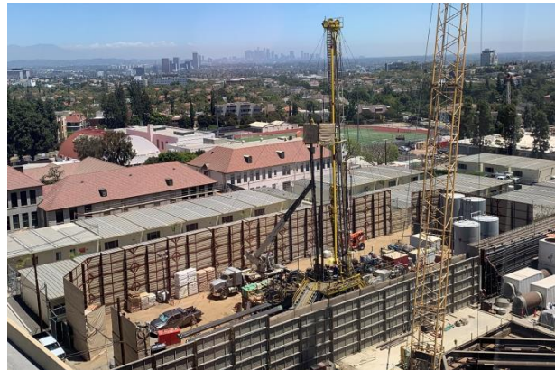
Oil Well Abandonment at Beverly Hills High School
