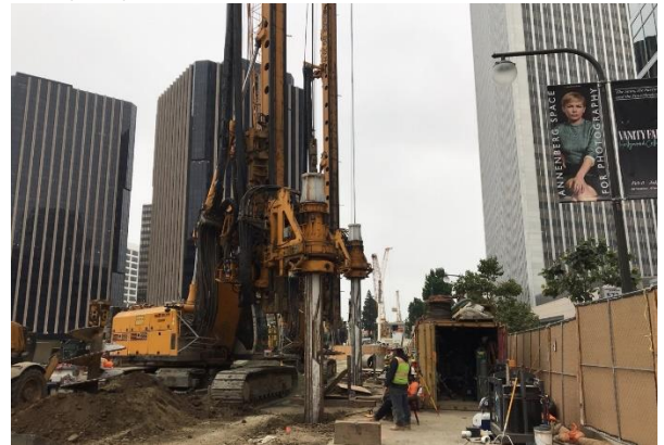
Pile Installation in Century City
