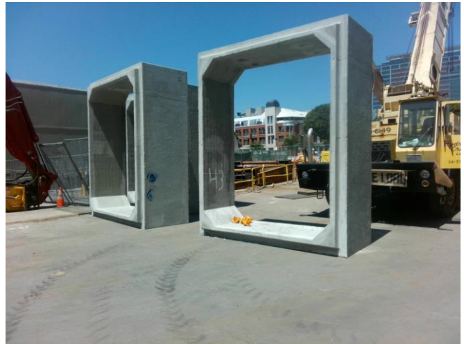
Reinforced Concrete Boxes for Storm Drain Relocation
