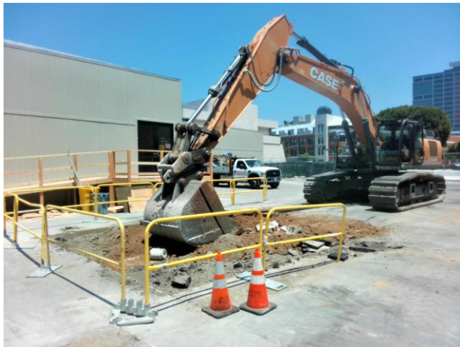
Asphalt Concrete Removal for Storm Drain Relocation
