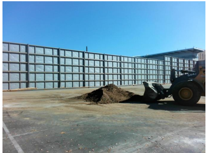
Spoils Removal after Sound Wall Assembly at Westwood/UCLA Staging Yard
