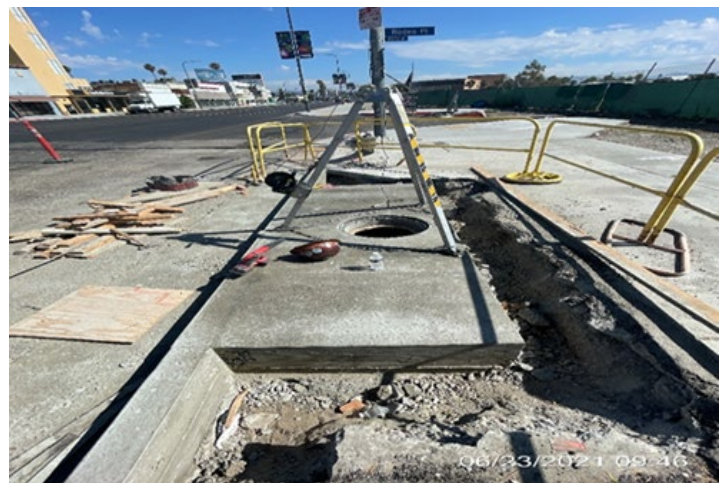
EXPO STATION SITE – Removing formwork from Catch Basin #11 on northbound Crenshaw Blvd and Rodeo Pl.
