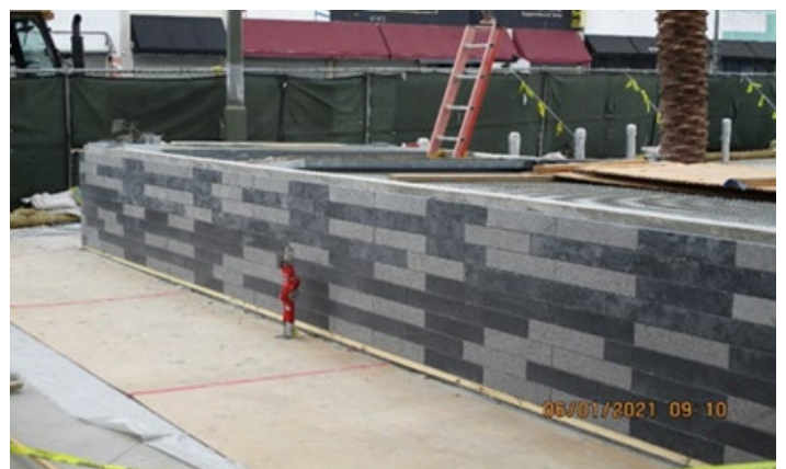
MLK STATION – Continue granite tile installation to the exterior walls of the Fresh Air Intake Shaft 2.
