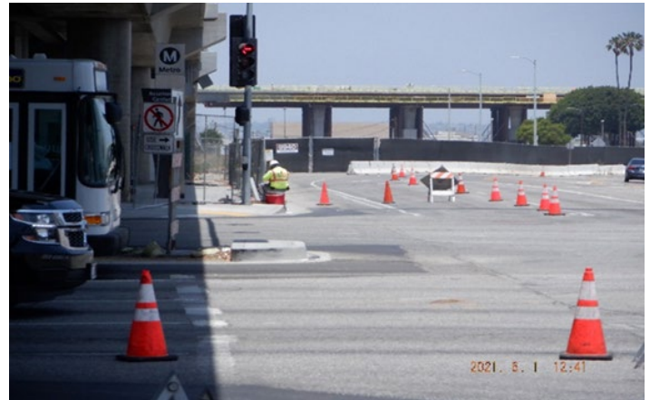
AVIATION/CENTURY STATION – STA 68+50 looking north – Aviation/Century Street lighting work by DB Electric
