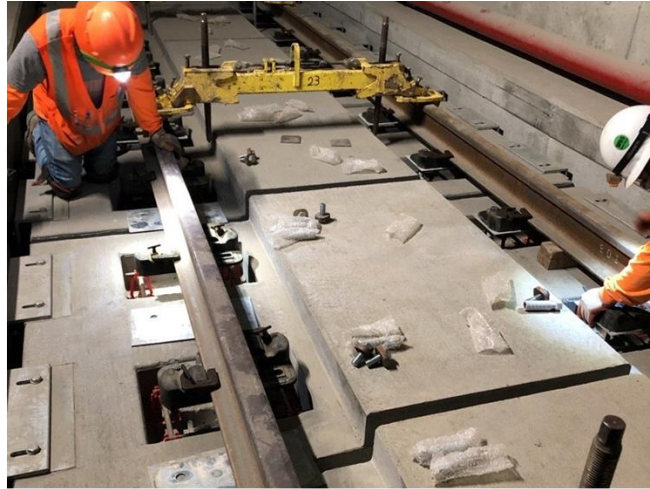
Installation of DFT pad assembly in tunnel
