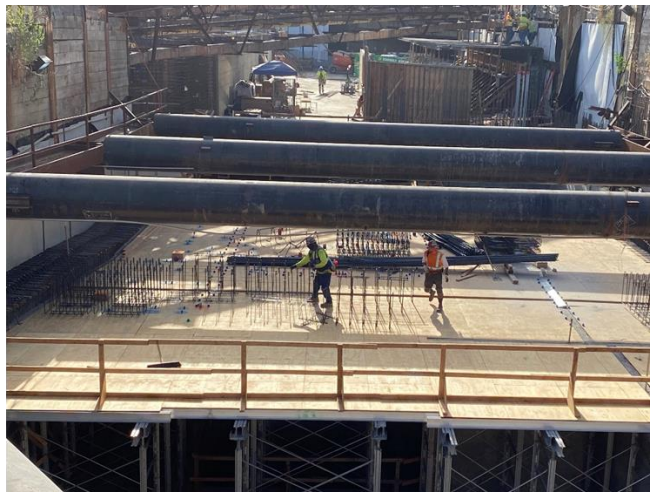
Rebar installation at roof level deck at Grand Av Arts/Bunker Hill Station
