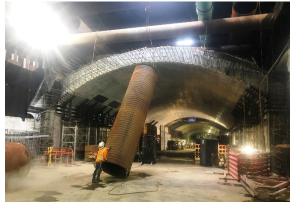
Wilshire/La Brea Station Arched Roof
