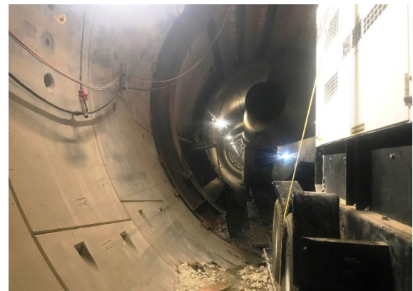
Reach 1 Cross Passage #8 Saw Cutting
