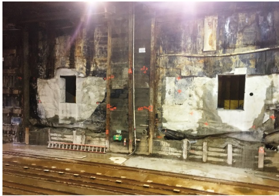
Existing Knockout Panel at Western Interface Chamber
