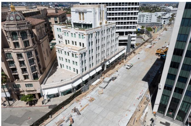
Wilshire Blvd. Decking During the Temporary Full Street Closure
