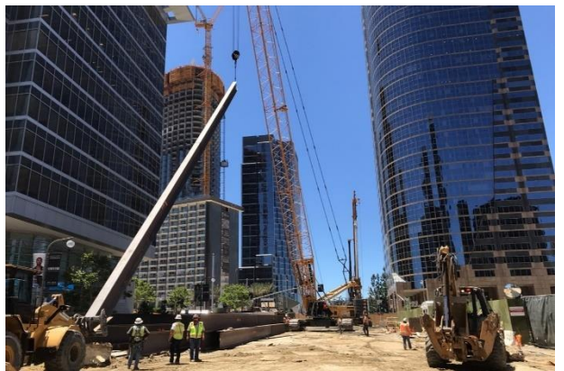
Pile Installation in Century City
