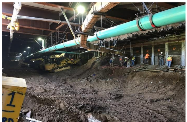
Wilshire/Rodeo Station Excavation Activities
