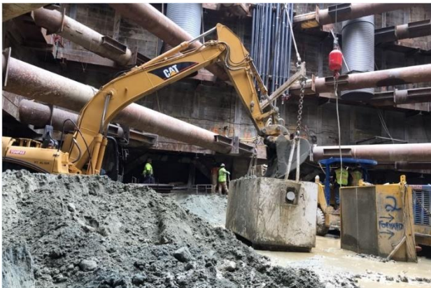
Tunnel Access Shaft Excavation Activities in Century City
