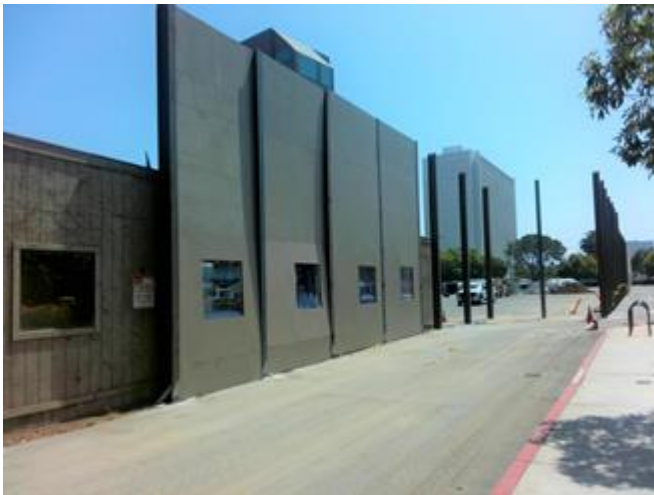
Temporary Sound Wall Barrier at Westwood/UCLA Staging Yard
