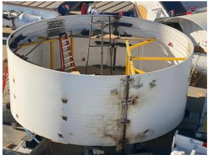
TBM Shield at VA
