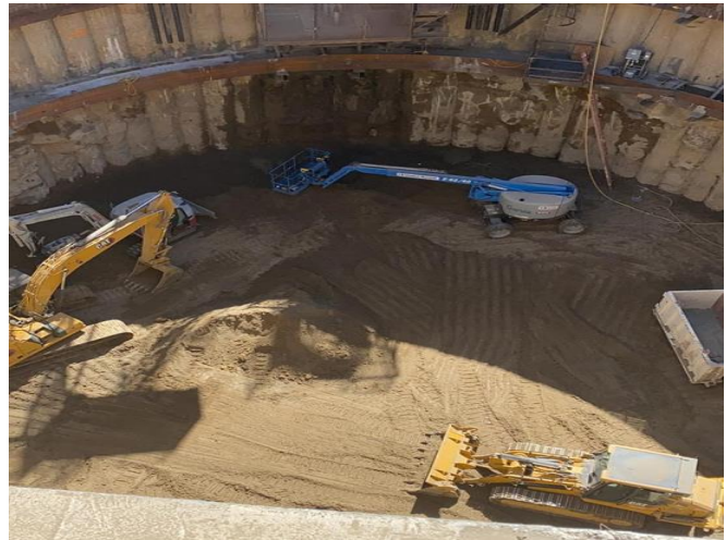
TBM Launch Shaft Excavation
