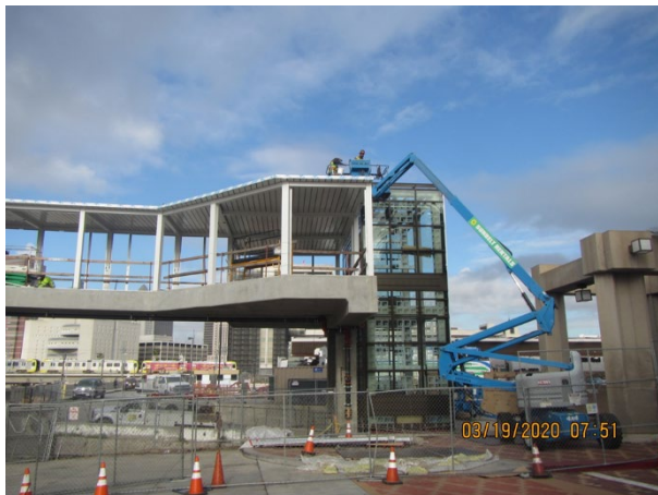
Installation of elevator outside glass
