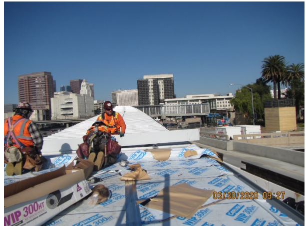
Installation of Pedestrian Walkway roof
