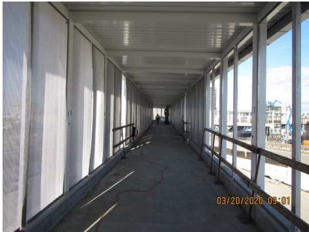
Stainless steel panels on Ped Bridge and Walkway
