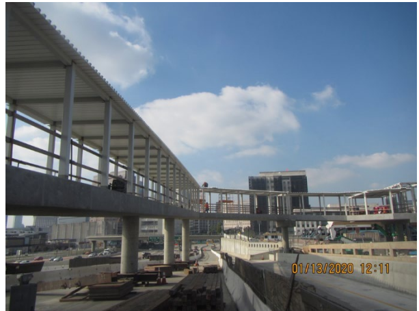
Installation of metal roof deck
