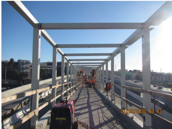
Pedestrian Bridge: Erecting structural steel
