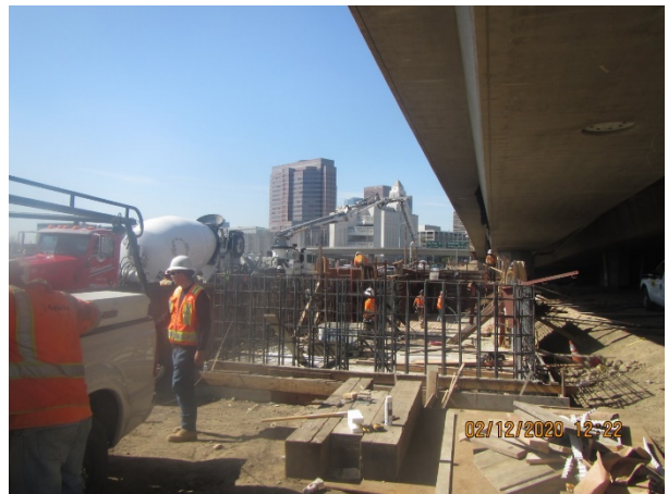
Austin Vault: Rebar installation and pouring concrete
