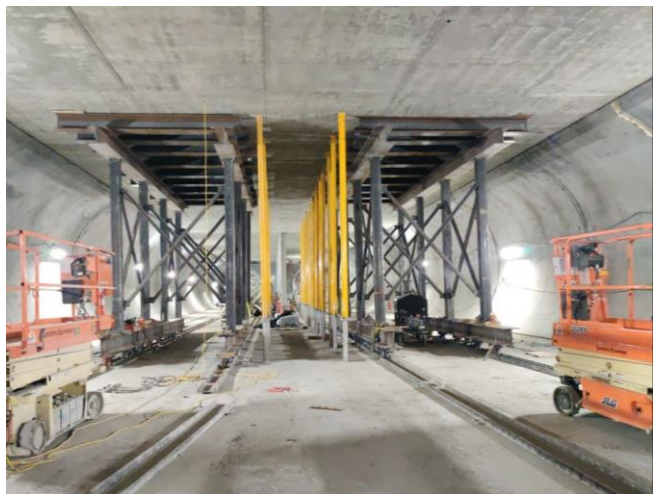
Crossover Cavern overview
