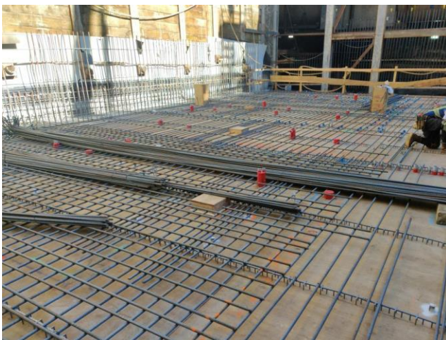
Rebar installation at the entrance structure at Historic Broadway Station
