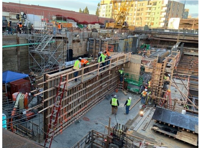
Interior wall placement in the future Little Tokyo/Arts District Station
