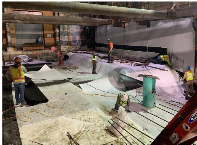
HDPE installation for invert at 7th/Flower
