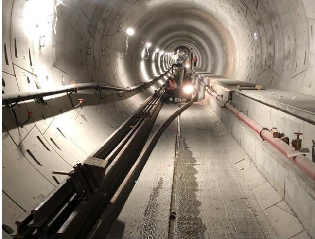
Staging Continuous Welded Rail (CWR) in bored tunnel
