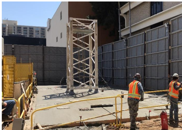
Tower Crane Foundation at the Tunnel Access Shaft in Century City
