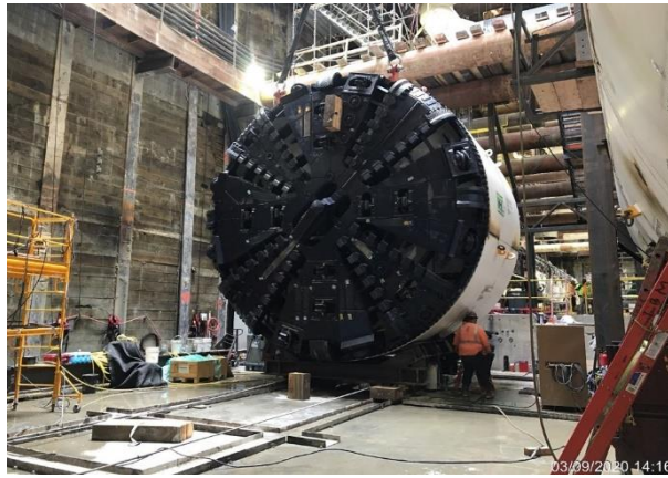
TBM Assembly at the Launch Box in Century City
