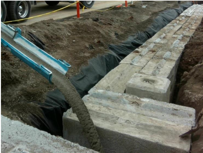
Slurry Backfill Between Concrete Blocks and Excavation at VA
