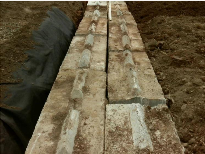
Placing of Concrete Block Wall Around Staging Area Roadway at VA
