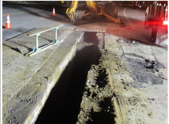
SCE Excavation of Line F
