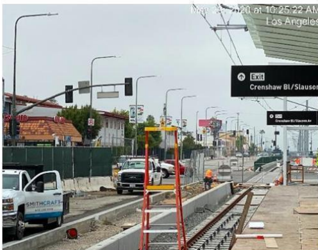
Hyde Park Station – Began signage installation at the platform level.
