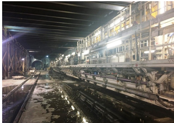
Purple TBM Mining Westward from Wilshire/Fairfax Station
