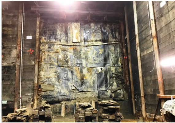
Existing Knockout Panel at Western Interface Chamber
