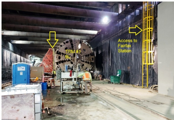
Red TBM at Wilshire/Fairfax Station
