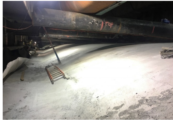
Finished Roof Concrete at Wilshire/La Brea Station
