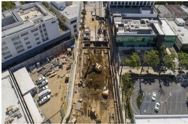
Tunnel Access Shaft in Century City
