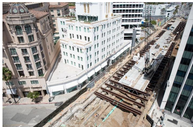
Wilshire/Rodeo Station Pile Installation and Decking During the Temporary Full Street Closure
