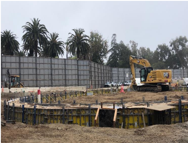
Collar Beam Formwork Removal at TTES
