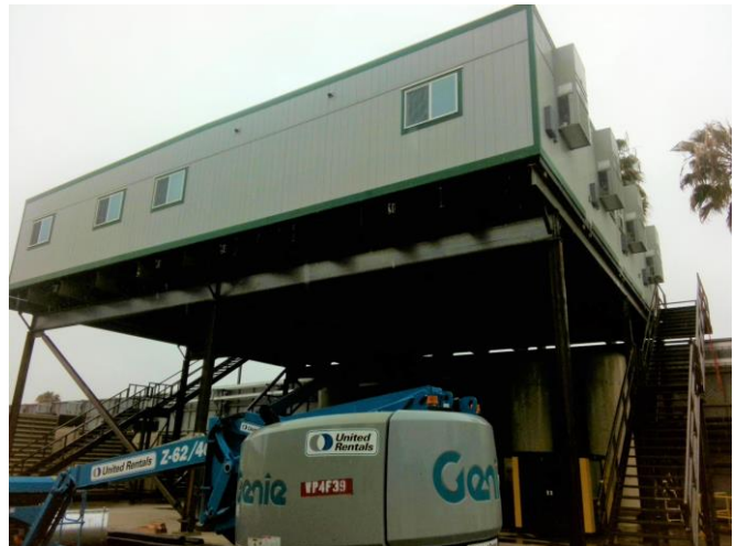
Modular Office Trailers Installation at VA
