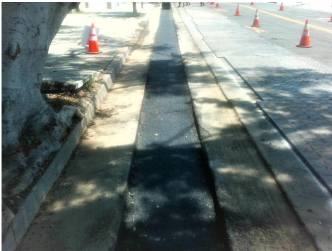
SCE Line B Paving on Federal Avenue
