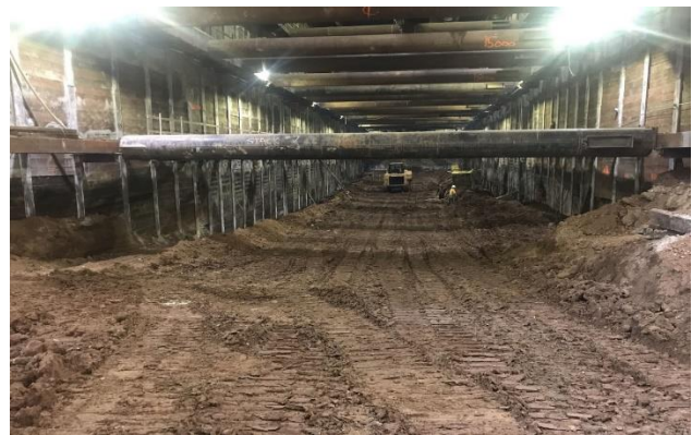
Wilshire/Rodeo Station Excavation Activities
