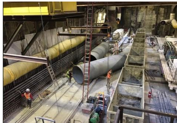
TBM Launch Box in Century City
