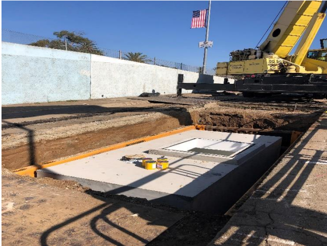
SCE Duct Bank Vault Installation along Wilshire Ramp near VA
