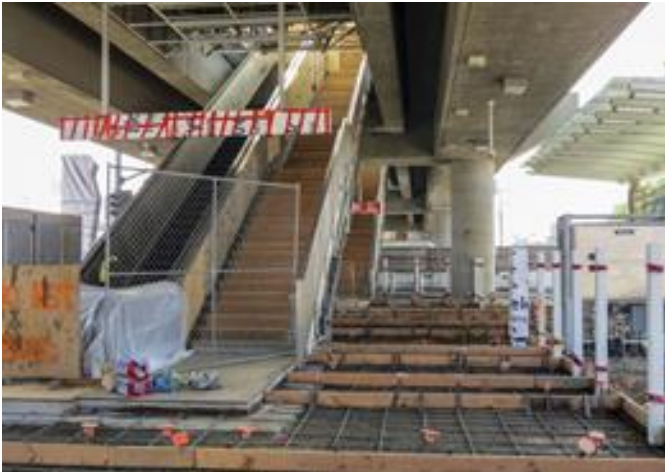
Aviation Century Station – ready for concrete placement of plaza floor.
