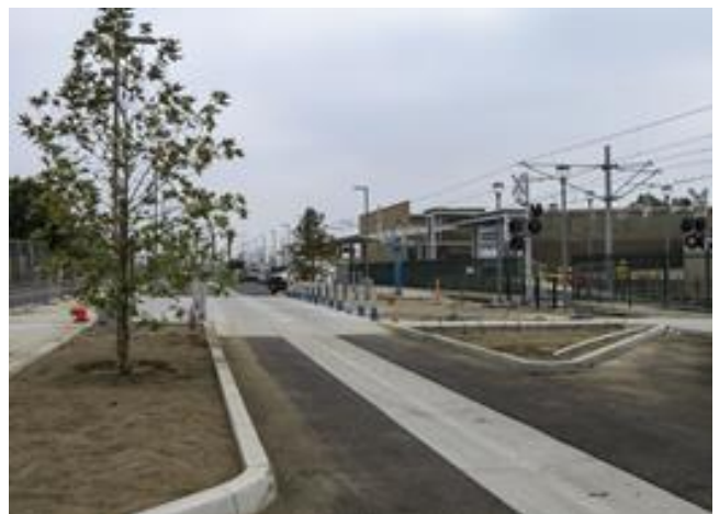
Fairview Heights Station – parking, landscaping and pedestrian Crossing..
