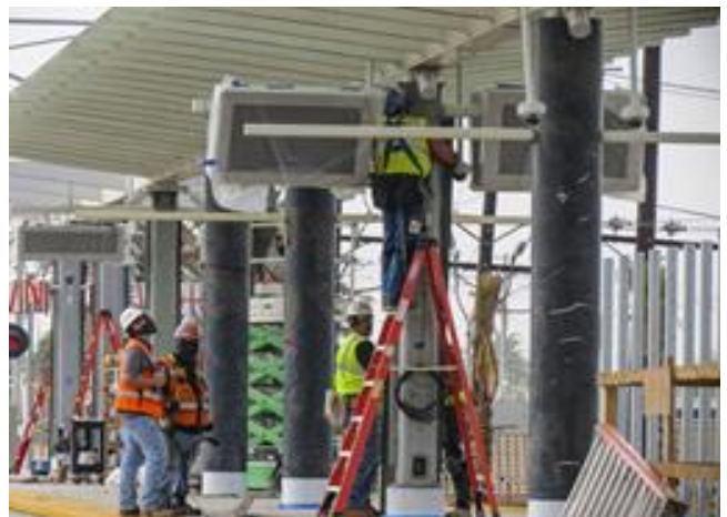
Downtown Inglewood Station – crews installing the platform LCD Message screen.
