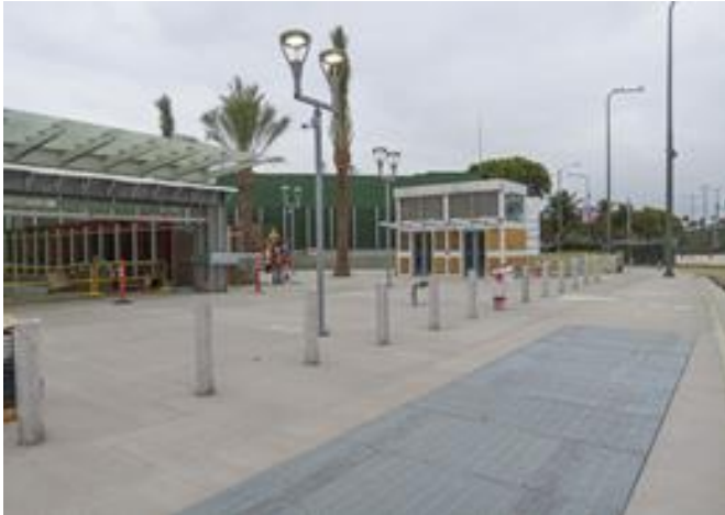
Leimert Park Station – plaza, lighting, landscaping, bollards, elevator and main entrance.
