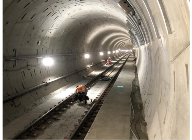
Stripping drain channel blockouts in Reach 1
