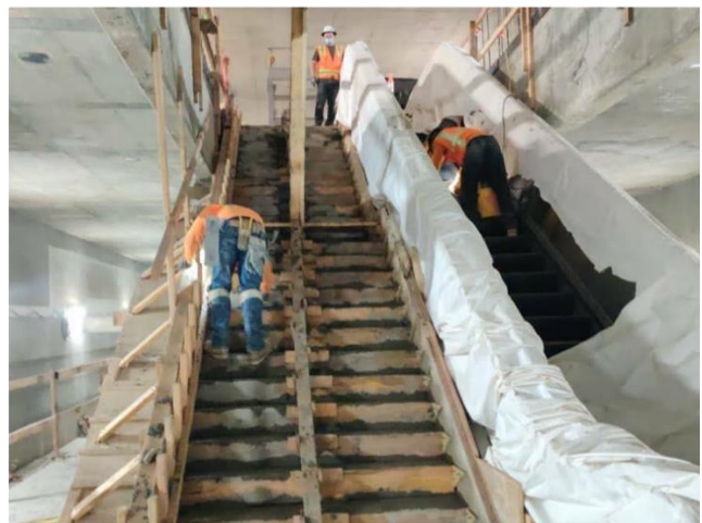
Concrete placement for platform stairs at Historic Broadway Station
