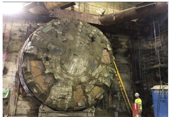
BR TBM "Harriett" Break-in to the Tunnel Access Shaft in Century City
