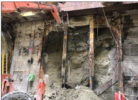
BR TBM "Harriett" Break-in to the Tunnel Access Shaft in Century City
