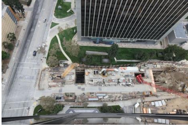
Aerial View of TBM Launch Box in Century City
