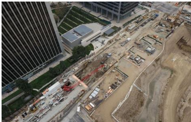
Excavation Activities West of the TBM Launch Box in Century City
