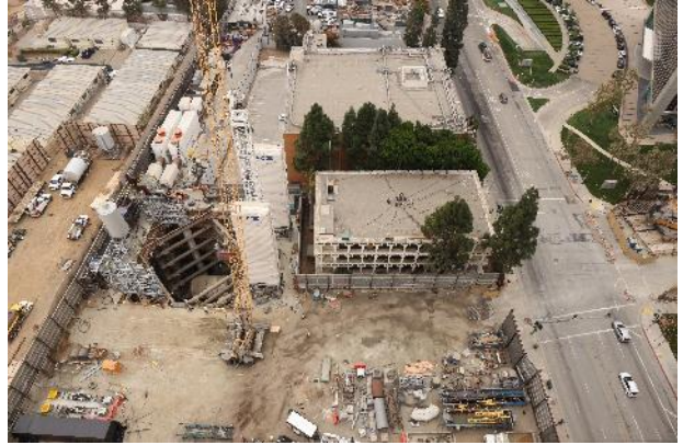
Aerial View of Tunnel Access Shaft in Century City
