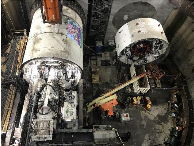
TBM Assembly at Tail Track Exit Shaft
