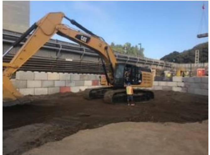
Excavation of the Temporary Muck Pit for Tunnel Excavation
