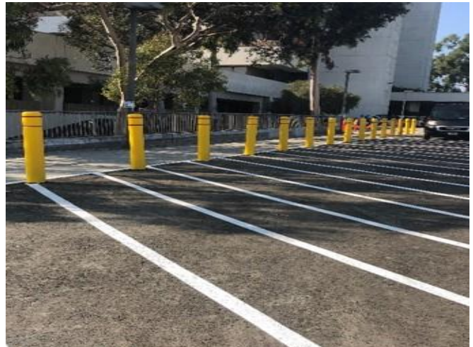
VA Parking Lot 43N Refurbishment
