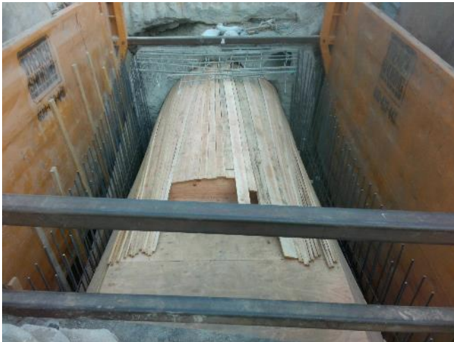
Stone Canyon Reinforced Concrete Box at UCLA Lot 36
