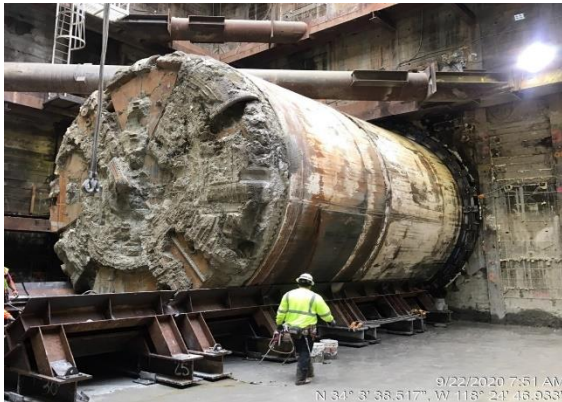
BL TBM "Ruth" Break-in to the Tunnel Access Shaft in Century City
