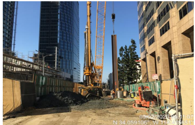
Pile Installation in Century City
