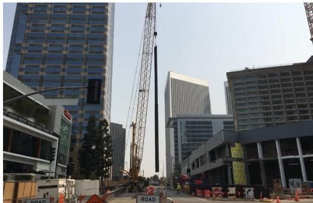
Pile Installation in Century City
