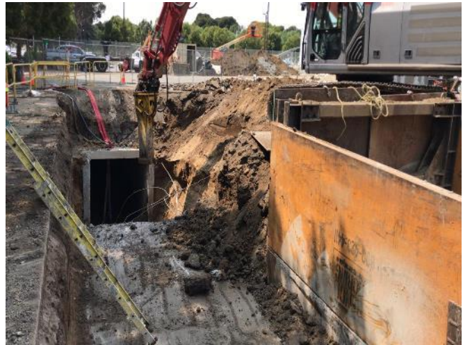
Demolition of Existing Storm Drain at UCLA Lot 36
