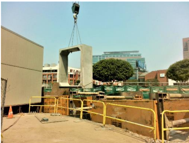
Reinforced Concrete Box Installation for Relocated Storm Drain at UCLA Lot 36
