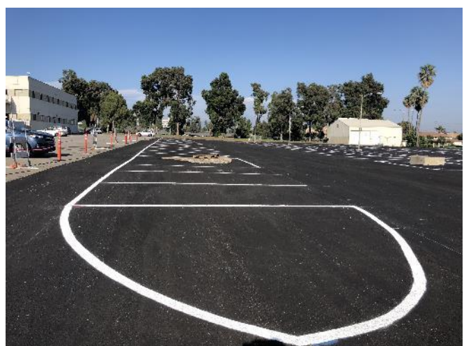
Striping and Parking Wheel Stops at VA Parking Lot
