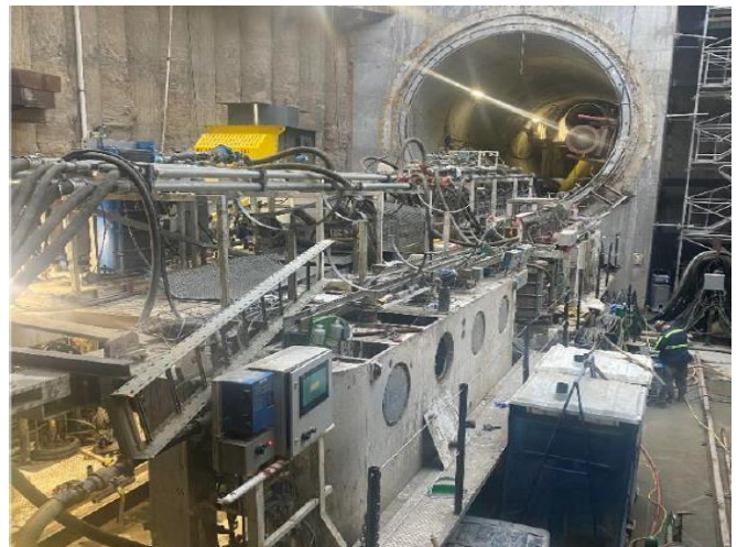
Tunnel Gantry Assembly at Tail Track Exit Shaft
