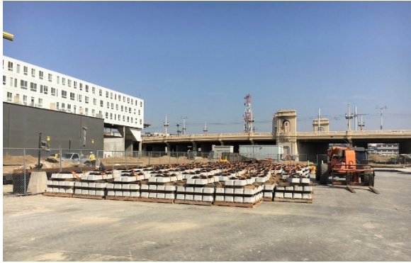
Track Block Delivery at the Division 20 Yard
