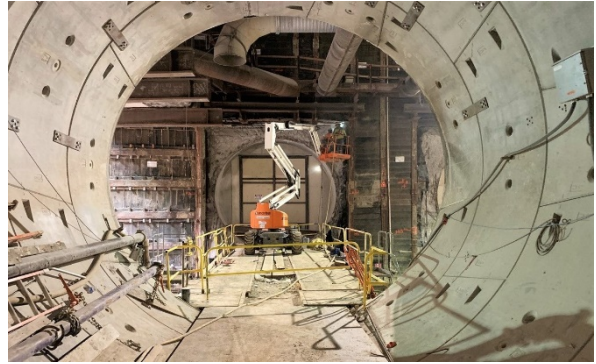
Removing Existing Concrete at Wilshire/Western Shaft
