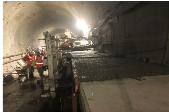
Reach 1 Tunnel Walkway Concrete Installation
