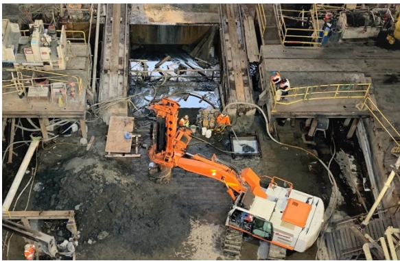
Elevator Casing Installation at Wilshire/La Brea Station
