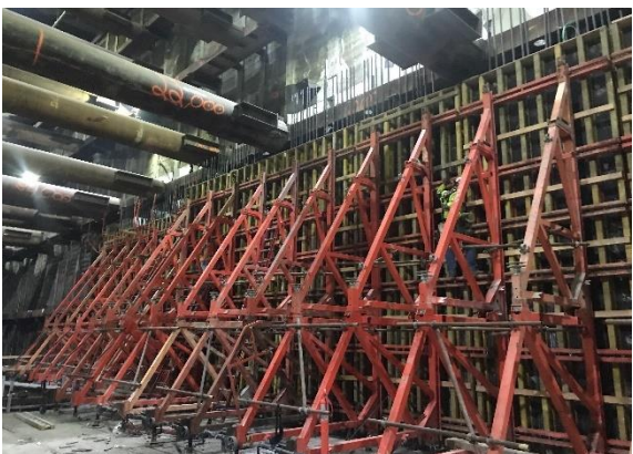
Concrete Placement for First Level Station Walls
