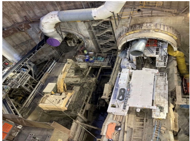
Aerial Overview at Tail Track Exit Shaft
