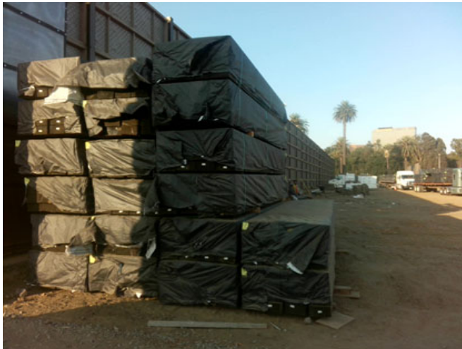
Lagging Delivered to Westwood/VA Station area (Lot 42)
