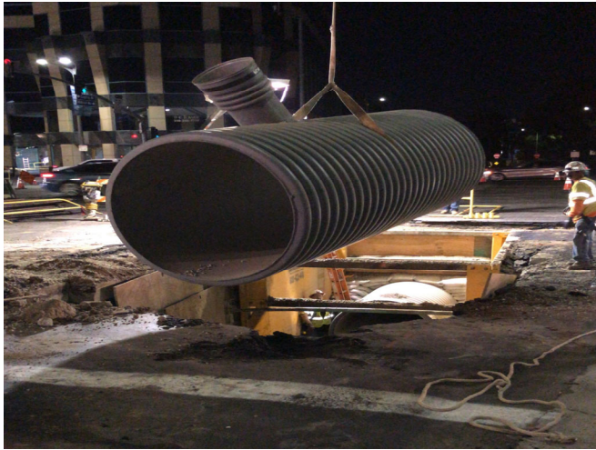
Sewer Relocation for Westwood/UCLA Station
