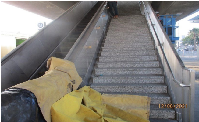
AVIATION STATION - Mounting the handrailing on the inside of the Aviation Station stairways. Facing south.
