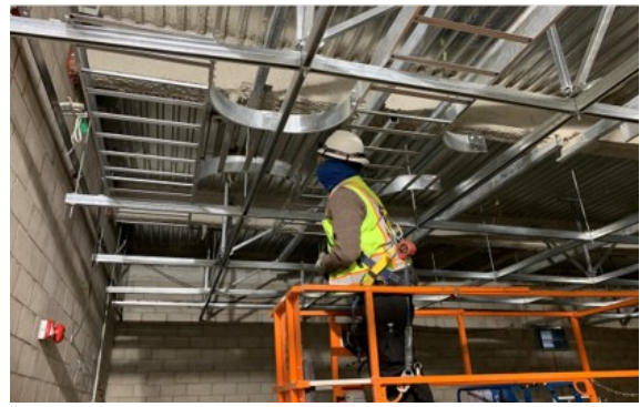
Installing Cable Trays at Wilshire/La Brea Station
