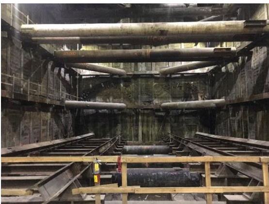
Tunnel Eyes, TBM Break-In (West)
