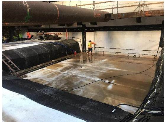
Waterproofing Membrane, Rebar and Formwork for Wilshire/Rodeo Station Entrance
