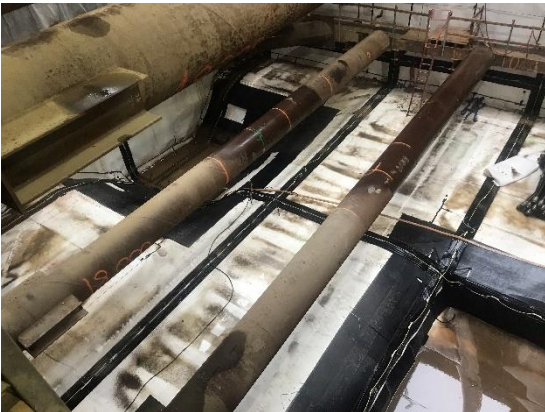
Waterproofing Membrane, Rebar and Formwork for Wilshire/Rodeo Station Entrance
