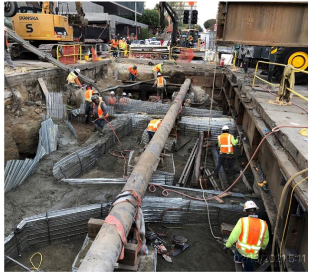
Backfilling of Broadway Closure
