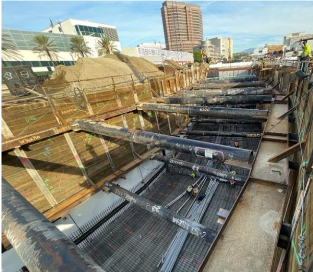
Alameda Cut & Cover rebar and MEP installation
