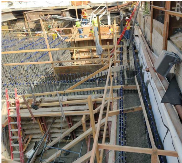
Entrance roof stem wall concrete placement
