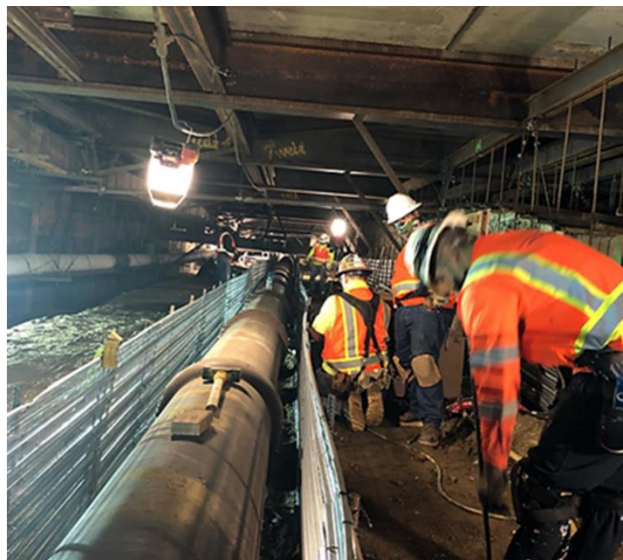
Stayform installation for 15" VCP sanitary sewer
