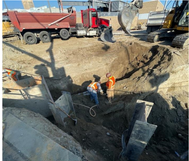
Excavation, lagging and exposing utilities at Temple St
