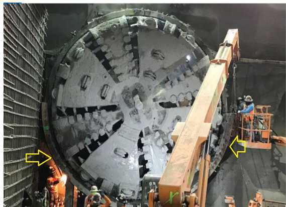
Purple TBM Arrival at Wilshire/La Cienega Station
