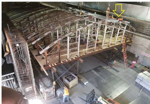
Roof Falsework Installation at Wilshire/Fairfax Station
