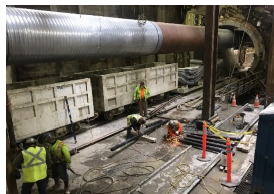
TBM Launch Box in Century City
