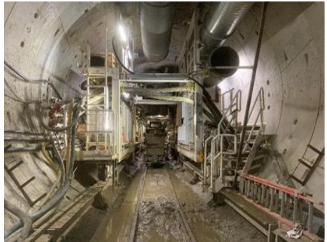
BR Tunnel Production Support Systems
