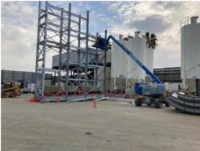
Assembly of the Belt Structure at Tail Track Exit Shaft
