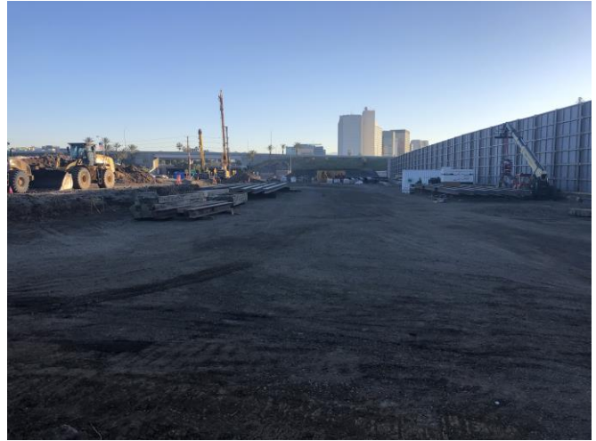
Staging Area at Westwood/VA Station
