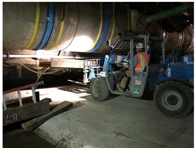
Water removal at East SOE Wall under Flower St
