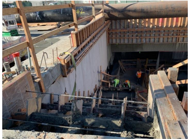
Concrete pour at future Little Tokyo/Arts District Station
