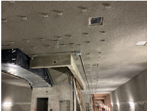
Pyrocl acoustical spray at Historic Broadway Station
